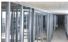
Drywall tracks to concrete and steel
