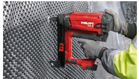
Light-duty applications in construction
