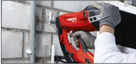
Conduits and light-duty pipes
