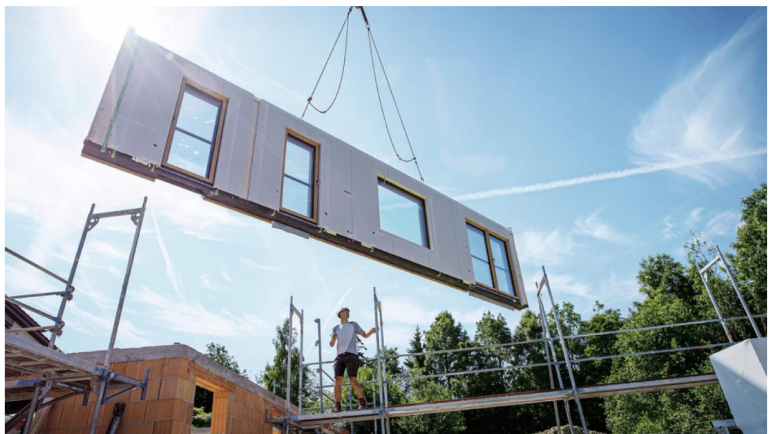
Fig. 2.5: Installation of a prefabricated timber panel on site
